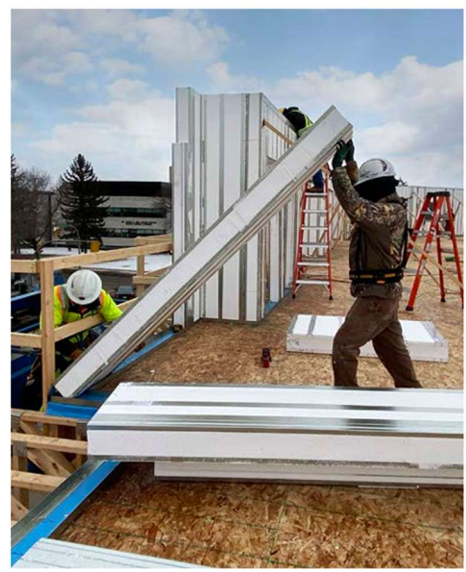
Greenstone Assembly Photos – Prefabricated panel assemblies add to construction speed and efficiency
