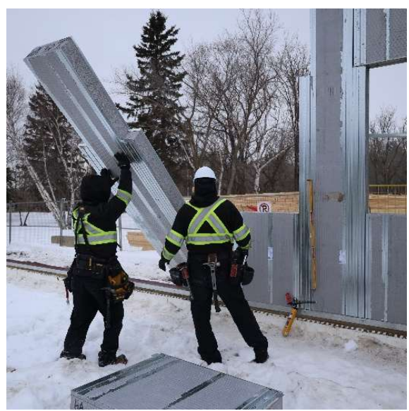
Greenstone Assembly Photos – Prefabricated panel assemblies add to construction speed and efficiency
